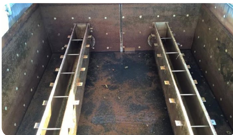
Figure 15. Appearance of the filter bed after a backwash at the follow up testing. Note the change in colour and reduction in surface mudballs and sludge on top of the filter. This is a significant improvement compared to Figure 12.
