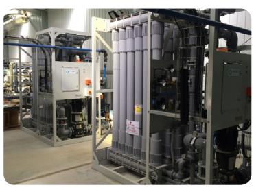
Taking into account TasWater's preferences and requirements, a WTP process design of raw water straining, dual train UF membranes, dual train NF membranes, pH/alkalinity adjustment via dual train calcite filters, dual train GAC adsorption, UV disinfection and chlorination was adopted.
