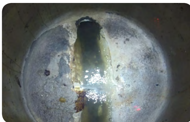
Figure 12. Still frame from SewCam footage from SP0208 maintenance hole with damaged benching. Black arrow indicates where SWI is entering from under the benching and into the channel.
