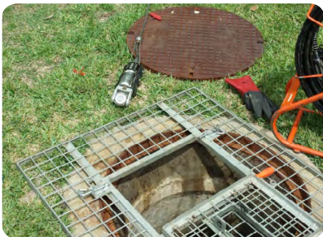
Figure 7. CCTV camera and tractor unit getting ready to be deployed into a maintenance hole. Unit is deployed into the sewer main and tractor unit is driven upstream or downstream looking for SWI sources entering the sewer main.
