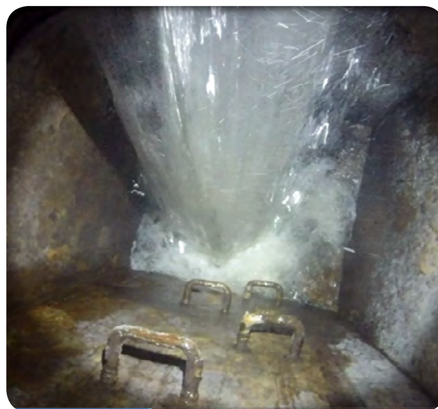
Figure 6. (Left) Still frame from SewCam footage of SP0011 collecting maintenance hole at low tide. (Right) Still frame from SewCam footage of the same maintenance hole at high tide showing SWI entering via the overflow window not visible in the frame.
