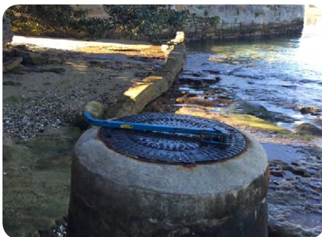
Figure 5. Accessible maintenance hole on harbour forshore. This can only be accessed during low tide as it is engulfed with tidal water at higher tides.
