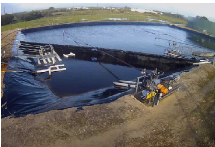
Figure 1A. The aerated pond wastewater treatment system at DBC during the anammox phase
