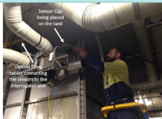
Figure 5. Installation of sensors set up in sewer.
