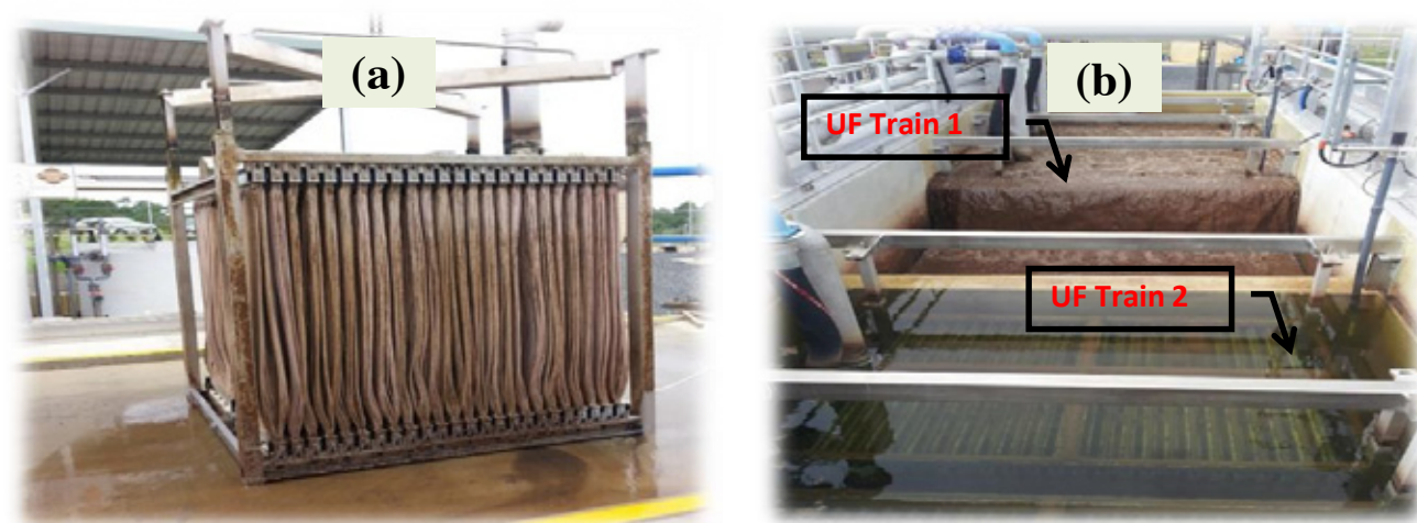
Figure 3. Membrane cassette a) removed for cleaning and b) soaked in NaOCl solution
