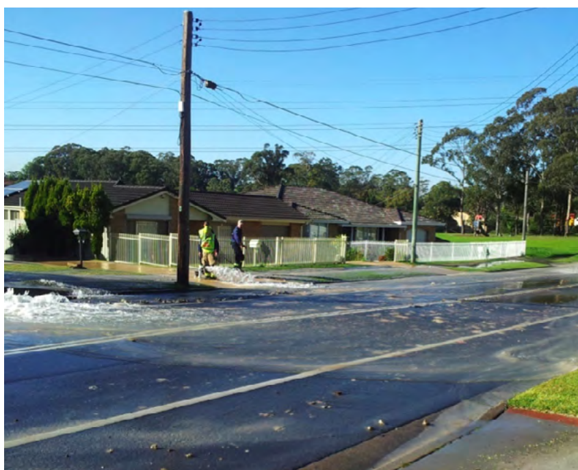
Figure 3. Photo of the result of a burst 100 mm watermain.
