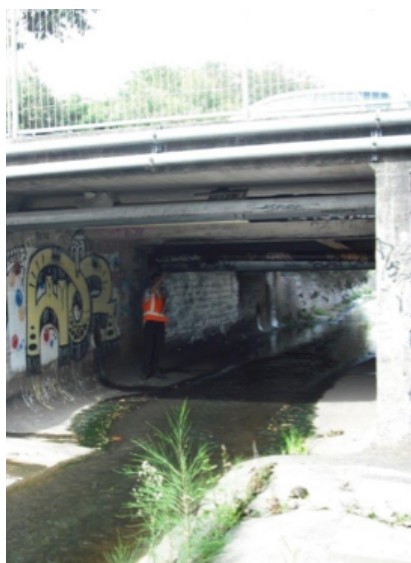
Figure 10. Existing Huntley St culverts showing the many intruding services
