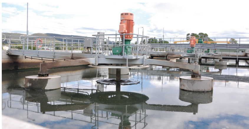
IDEA (intermittently decanted extended aerator) tank, with surface aerator.
