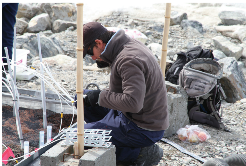
Figure 1. PRB installation to capture and treat hydrocarbon contamination from a diesel spill at Casey Station.
