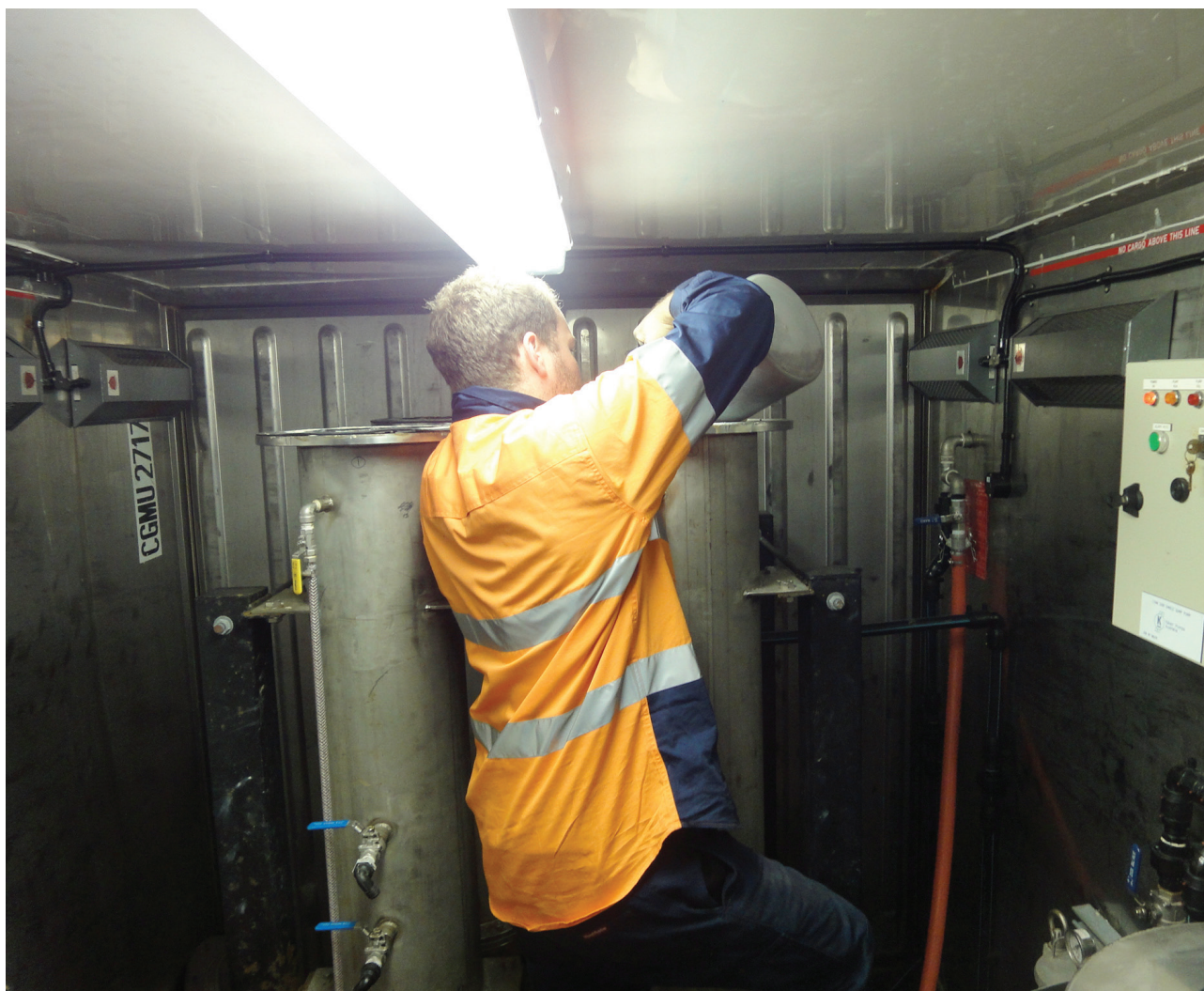
Figure 11. Filling the Casey WTP filters with carbon during the 2015–2016 summer season at Casey Station.
