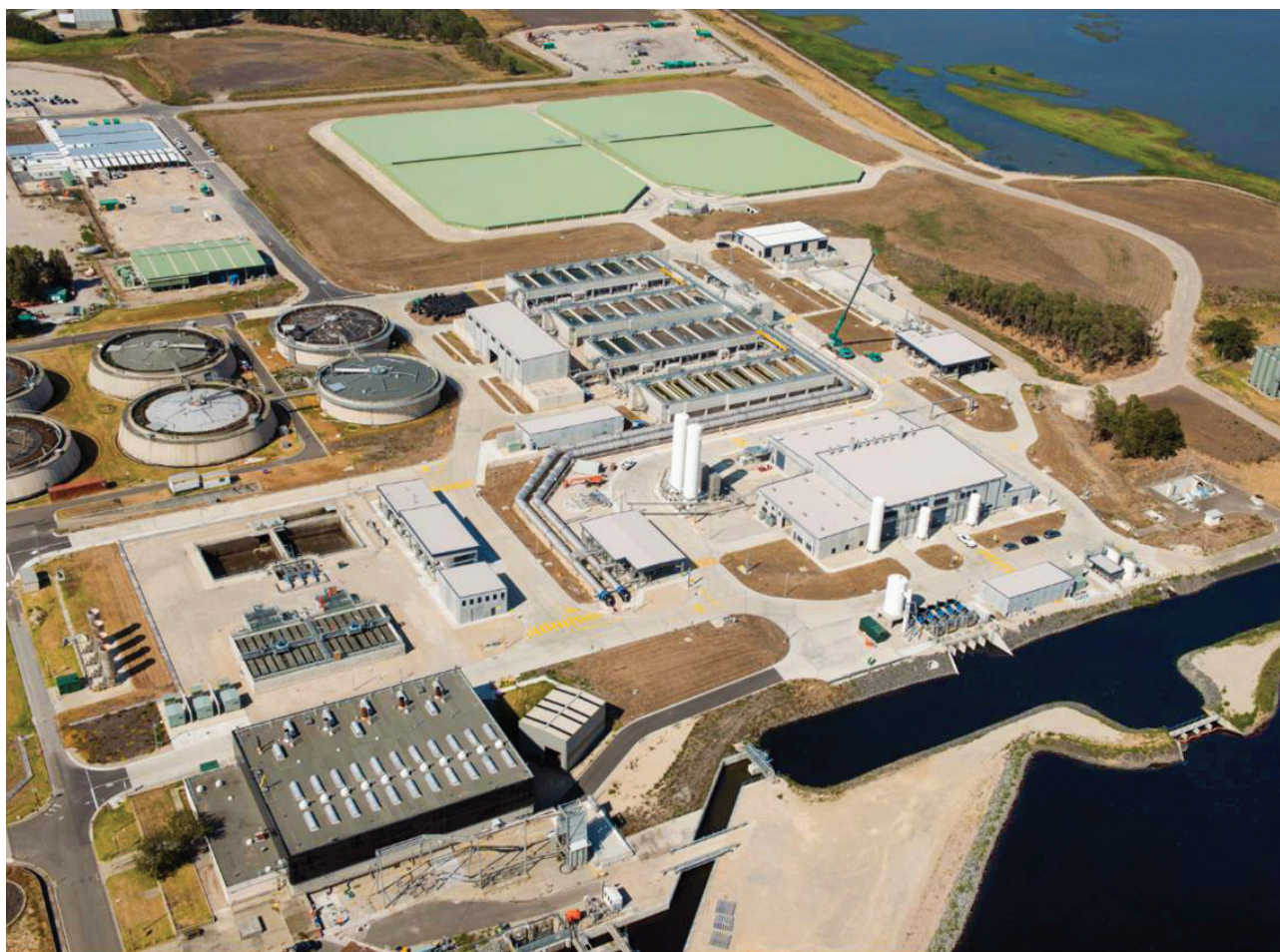
Tertiary treatment at Melbourne Water's Eastern Treatment Plant, 2012.
