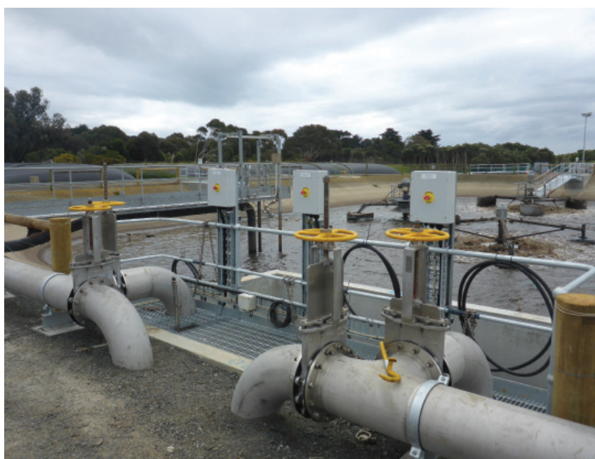
Figure 6. New mixed liquor (ML) pump station.
