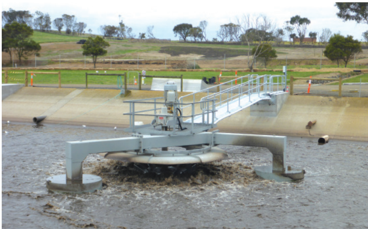
Figure 7. Surface aerator with new walkway.
