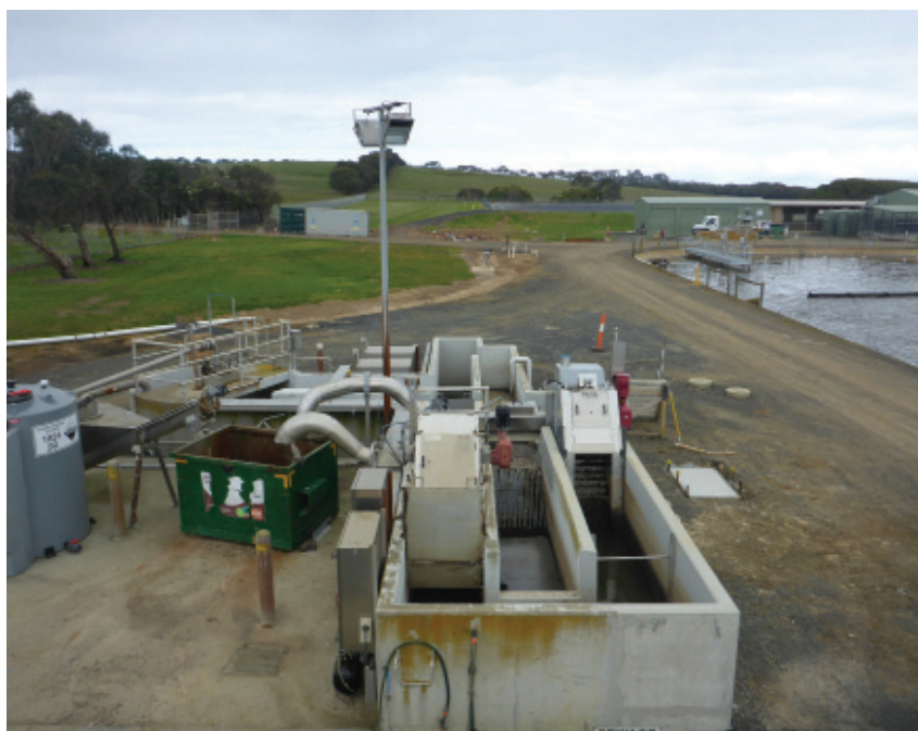
Figure 4. Inlet structure with new channel and new screen.
