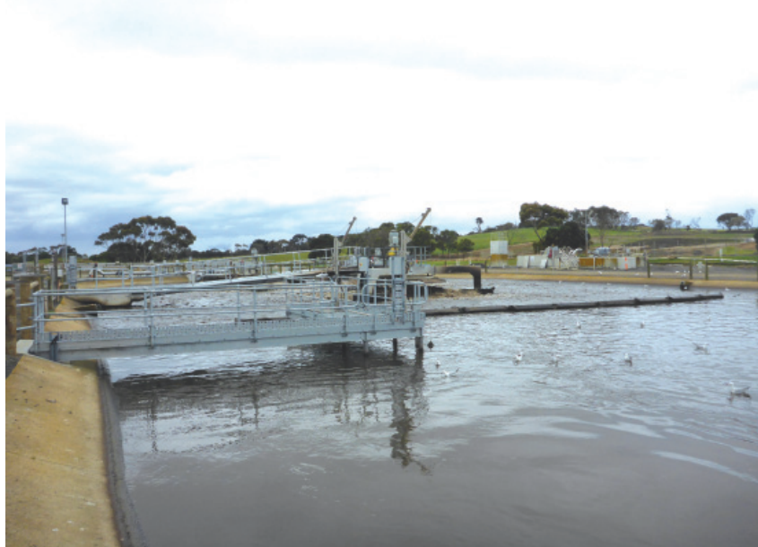
Figure 5. Bioreactor 1 anoxic zone.
