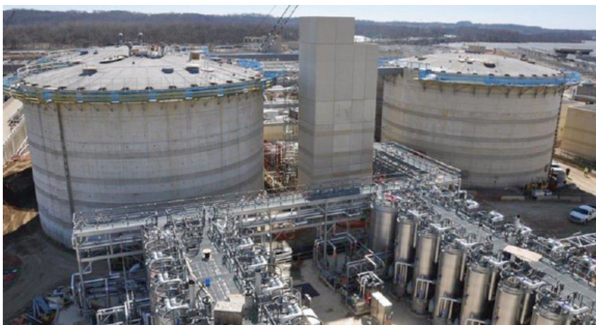
Figure 4. New thermal hydrolysis and mesophilic anaerobic digestion at Blue Plains AWTP.
