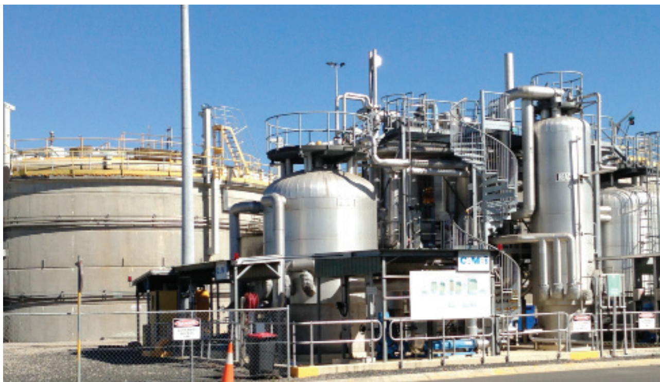
Figure 10. Oxley Creek CAMBI installation and digesters.
