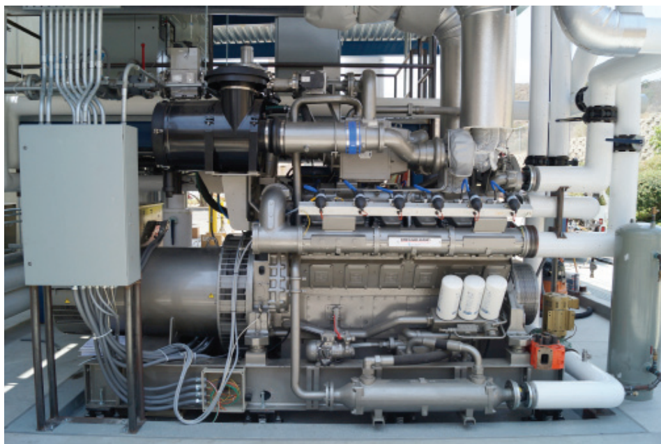
Figure 9. The 700 kW cogeneration unit installed in 2013.
