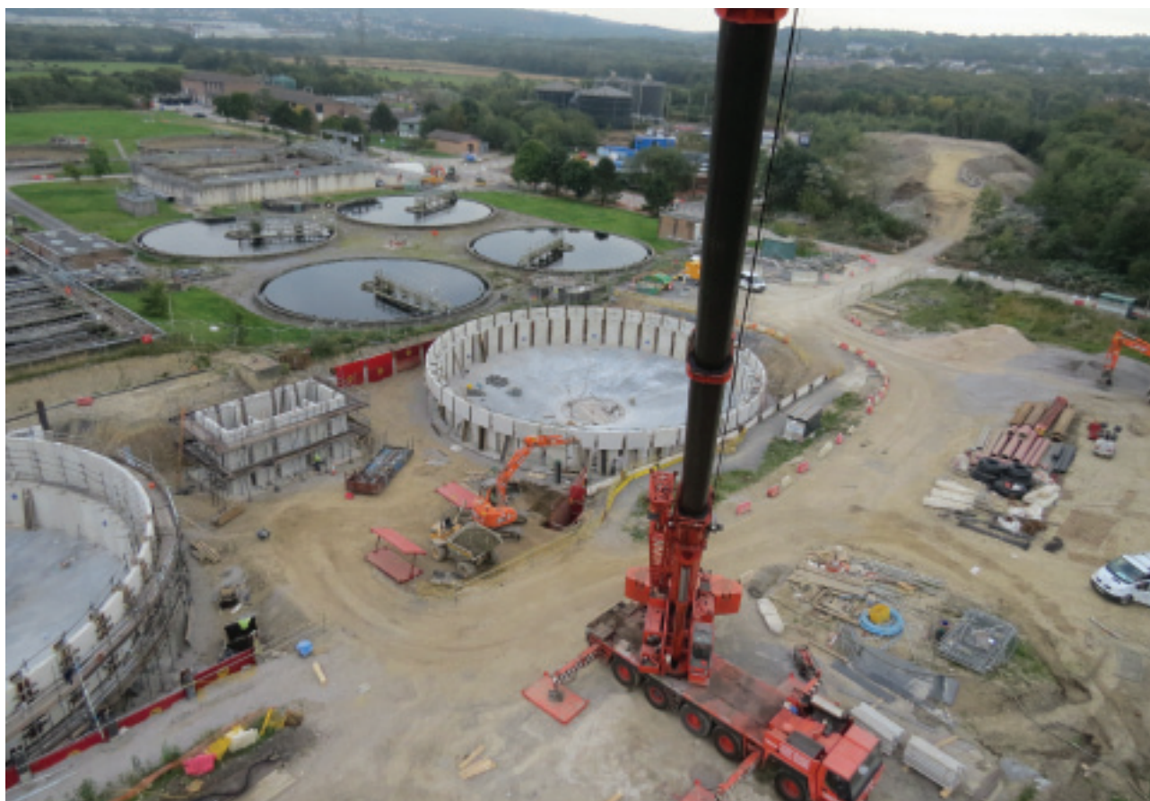
Figure 2. FST pre-cast wall sections at Gowerton WWTW by Carlow Precast.
