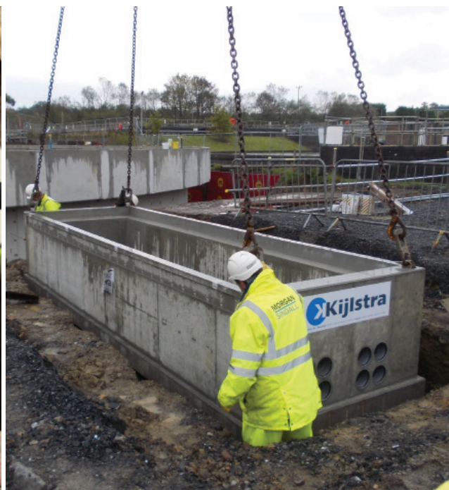
Figure 4. Kijlstra pre-cast MCC chamber being lifted into place at Gowerton WWTW.
