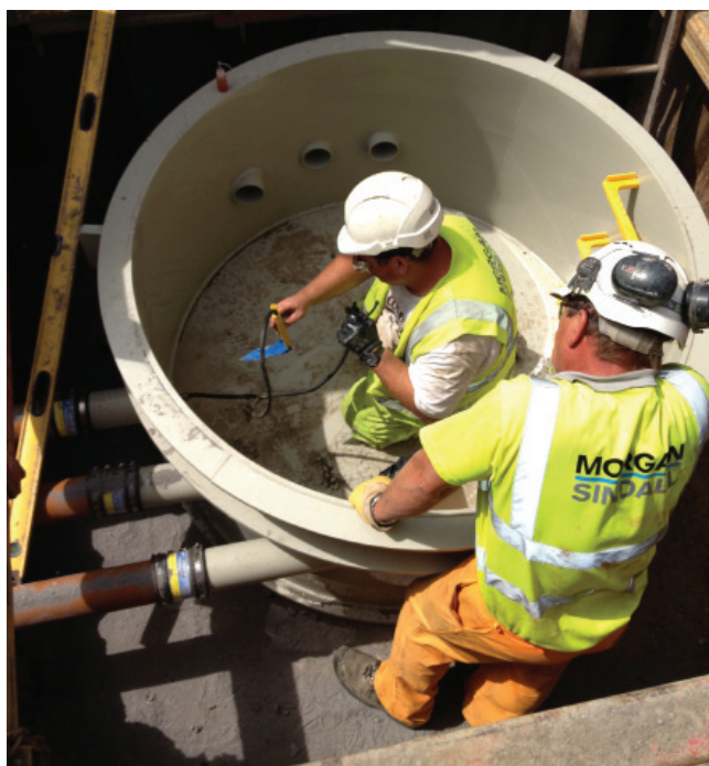
Figure 3. Pre-fabricated catchpit chambers by Pipex Px.
