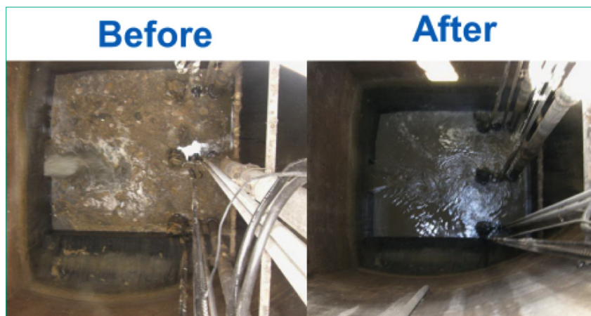
Figure 7. Before and after shot of the implementation of the auto-flush pump operating regimen.
