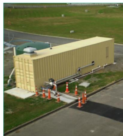
Figure 3. Recuperative thickener (RT) plant.
