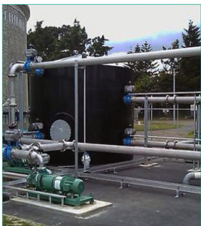
Figure 2. DAF sludge waste reception.
