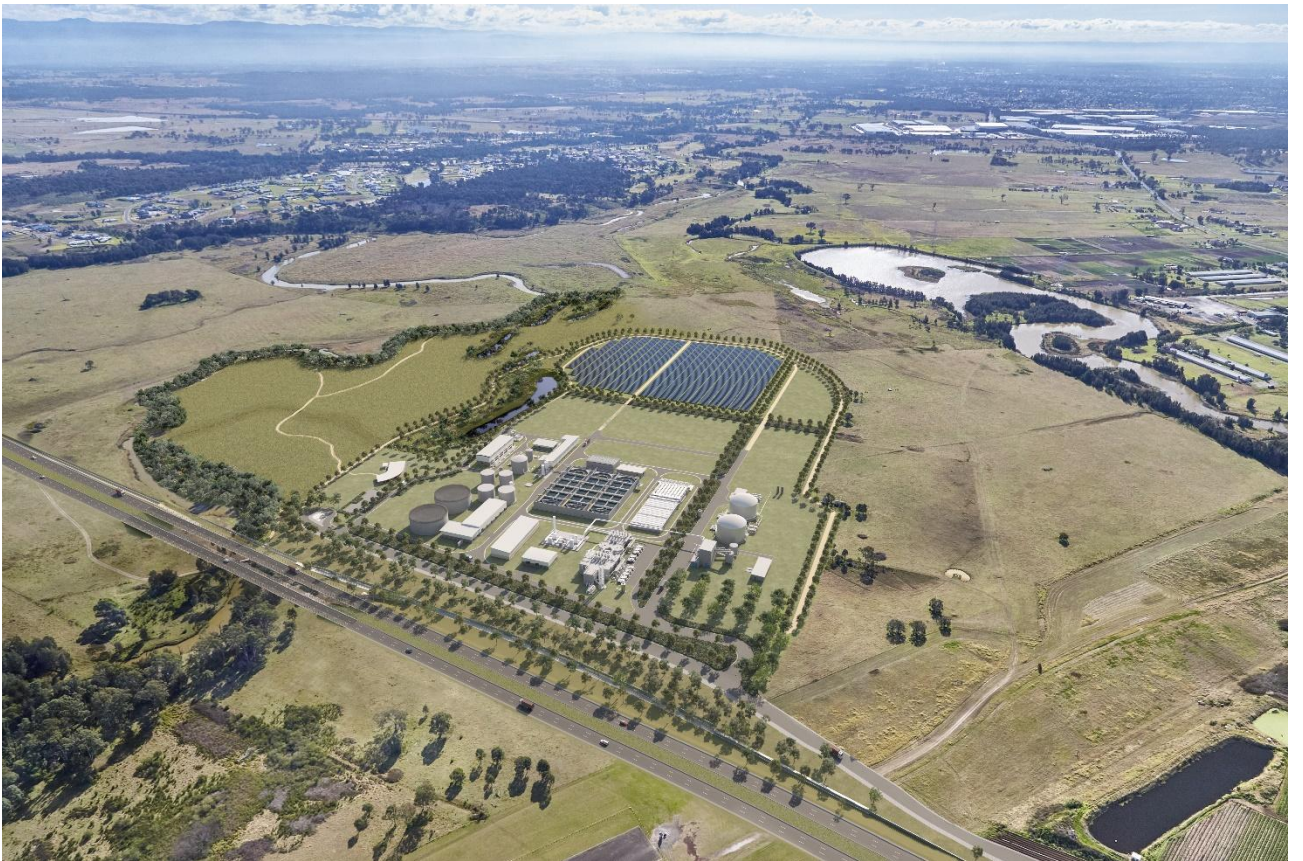
Figure 1: Upper South Creek AWRC Render (Stage 1 upgrade)
