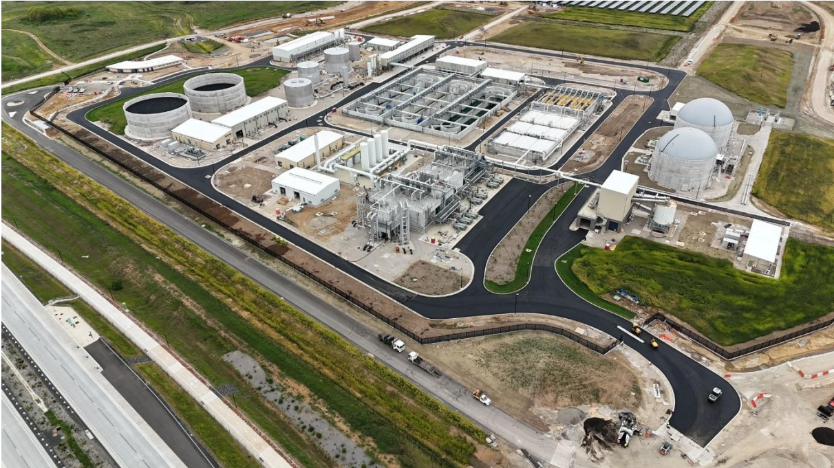
Figure 7: USC ARWC approaching the end of construction (February 2026)
