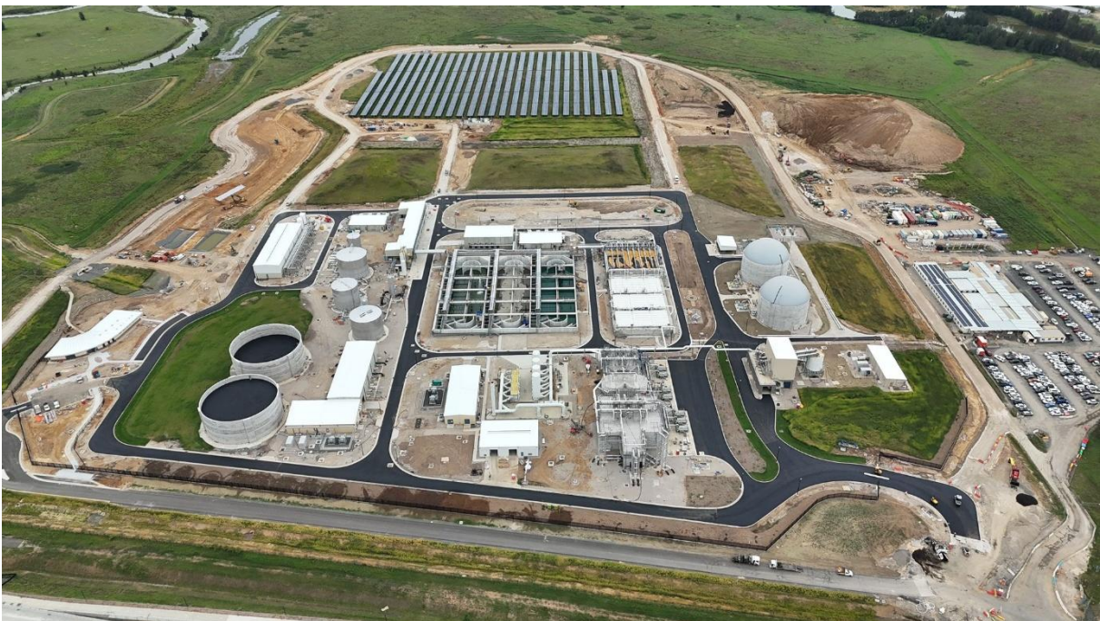
Figure 8: USC ARWC approaching the end of construction (February 2026)
