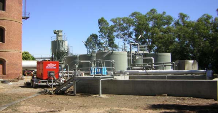
FLOOD equipment in use
