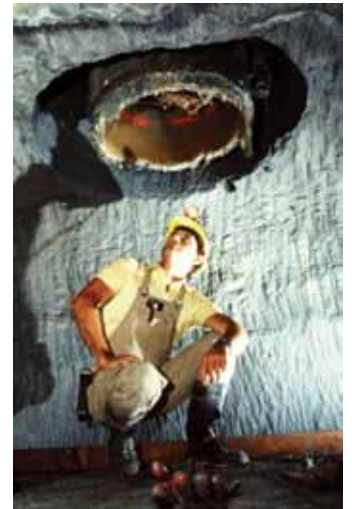
Image 9 - Sydney Water Board Employee - Graham Dixon - Crouching under Vertical Riser Shaft
