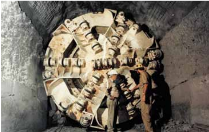
Image 5 - Tunnel Boring Machine
